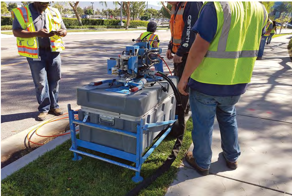
OntarioNet fiber is blown into existing conduit.
